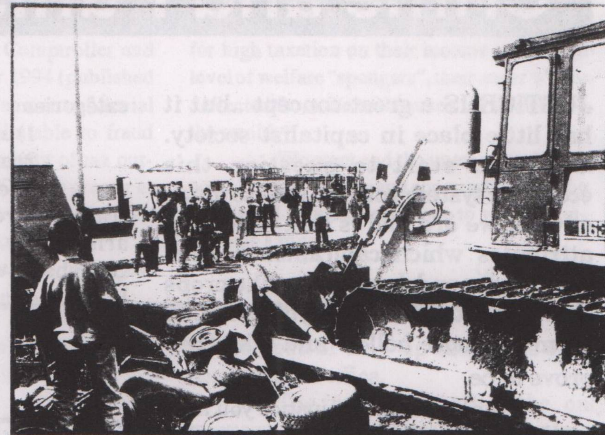
•Bulldozer being used to evict Travellers at Clondalkin
